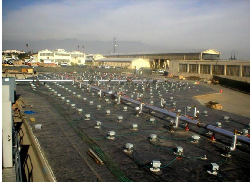
Picture 12: Full-scale ISTD operation on organic compounds contamination in the USA Source: Merly and Hube (2014)
