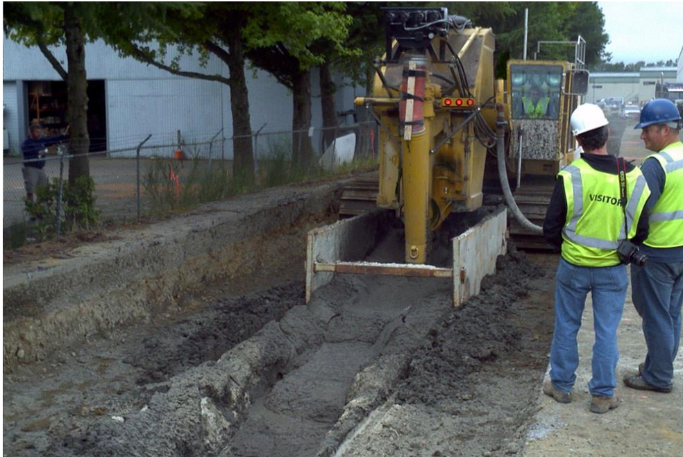
Picture 10: Combined trenching and slurry insertion
